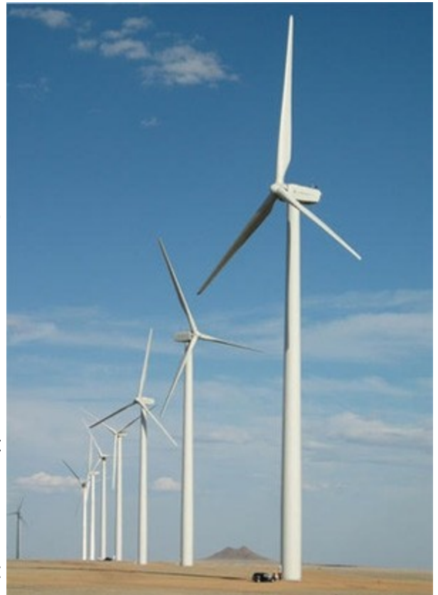
1.5 Megawatt General Electric wind turbines
